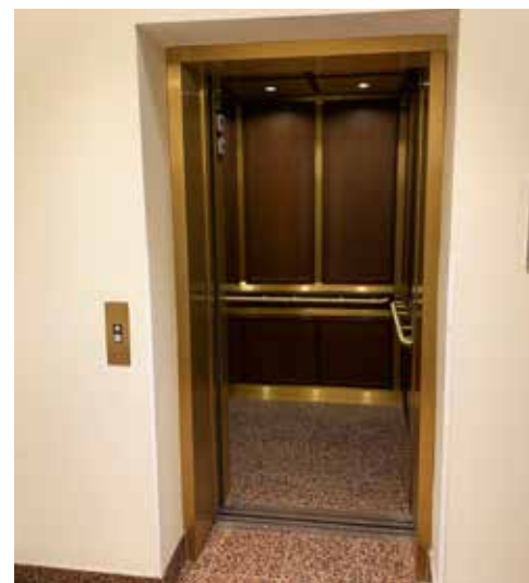
The elevator - still going strong after 25 years!
