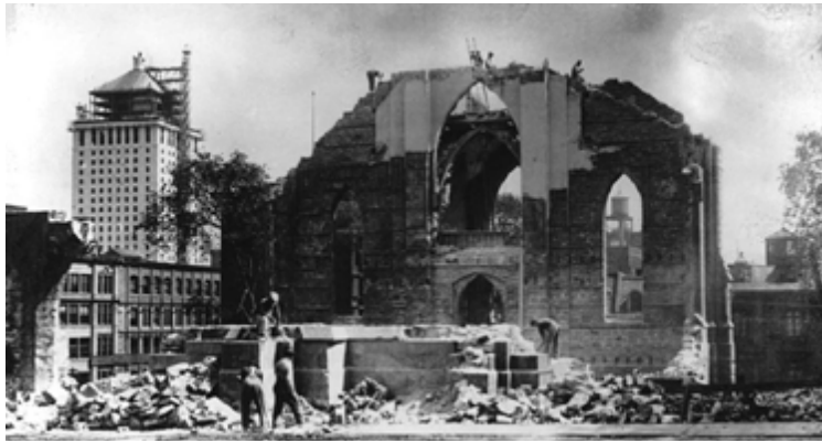
Demolition of St. Andrew's Church
